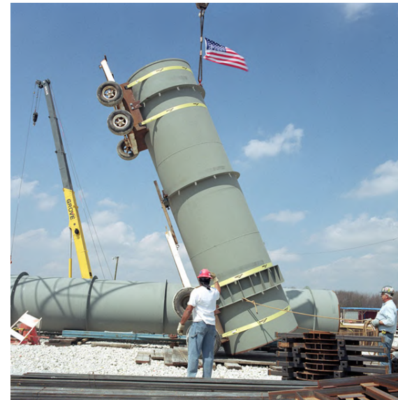
NuMI decay pipe ( \sim 1 Torr vacuum, length: 675 m)
