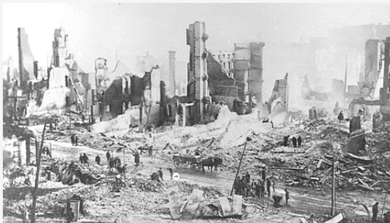
Fire, Baltimore 1904 - incompatible fire brigades' hydraulics from different cities NIST
